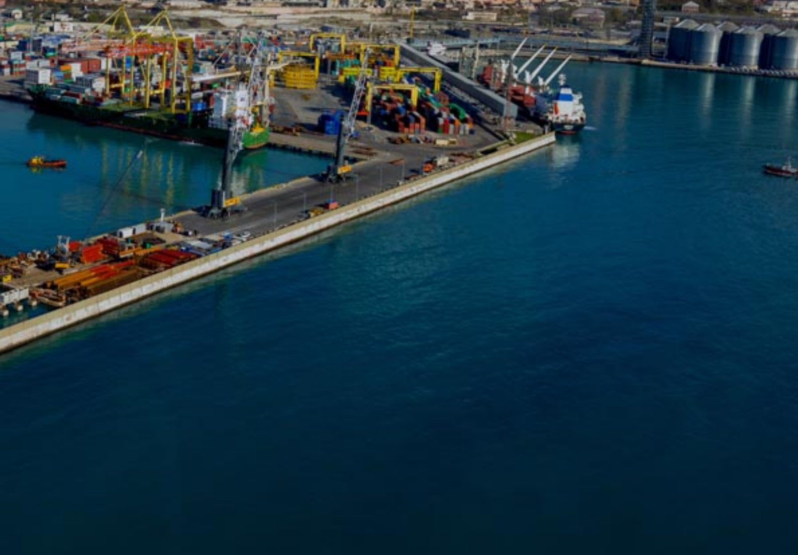
Halifax (Nova Scotia, Canada). Construction of Deepwater pier number 38. Photo credit: Ivan Studenov
