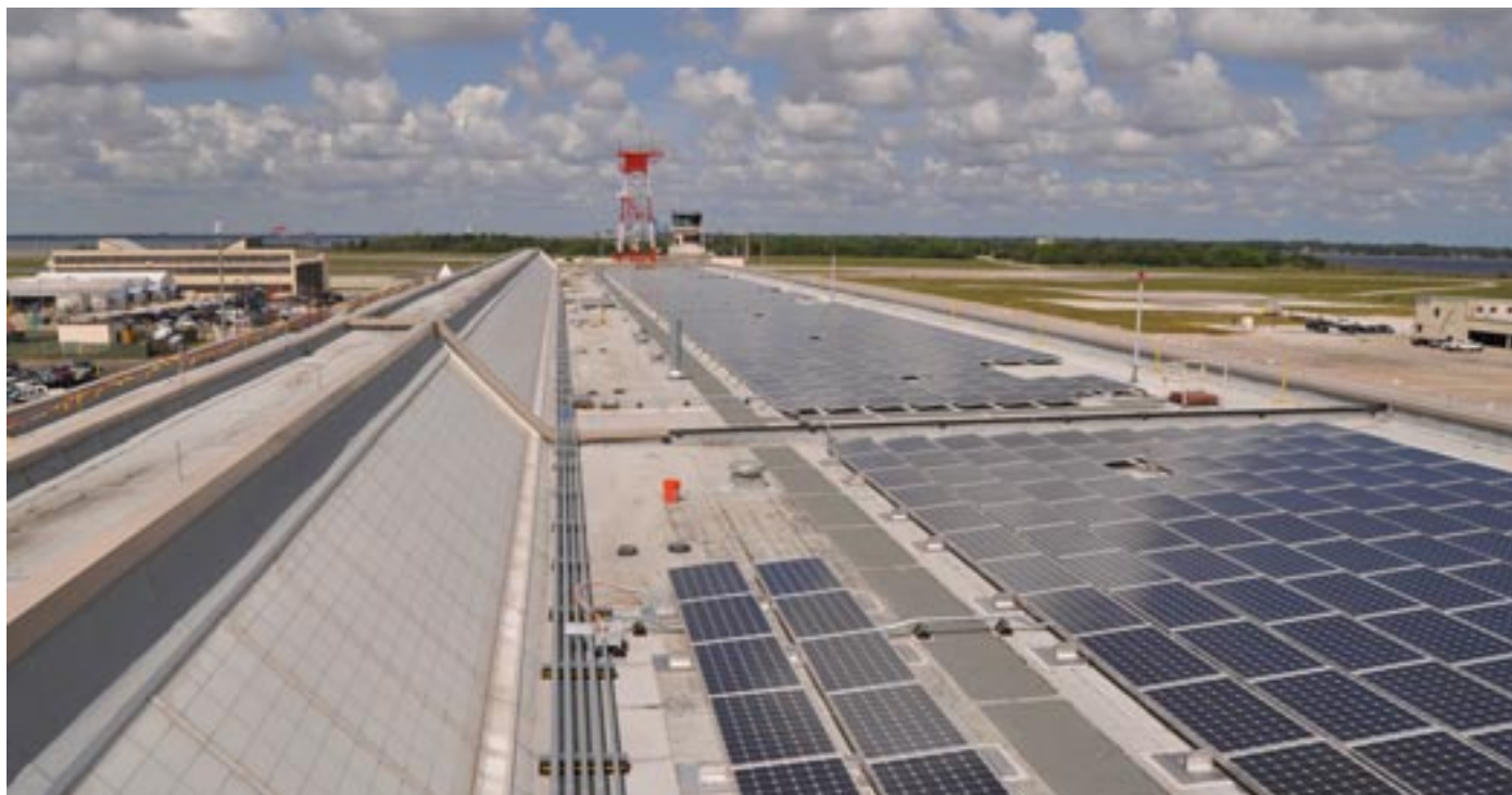
Some of the 2,534 solar photovoltaic (PV) panels installed on the roof of Naval Air Station Jacksonville's Hangar 1122 to help reduce the building's conventional energy usage and promote environmental sustainability. Photo by: U.S. Navy - Clark Pierce/Released
