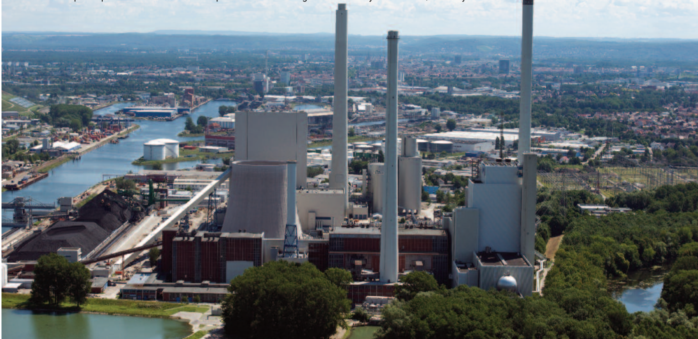
The RDK8 steam power plant at the Rheinhafen-Dampfkraftwerk electrical generation facility in Karlsruhe, Germany.
