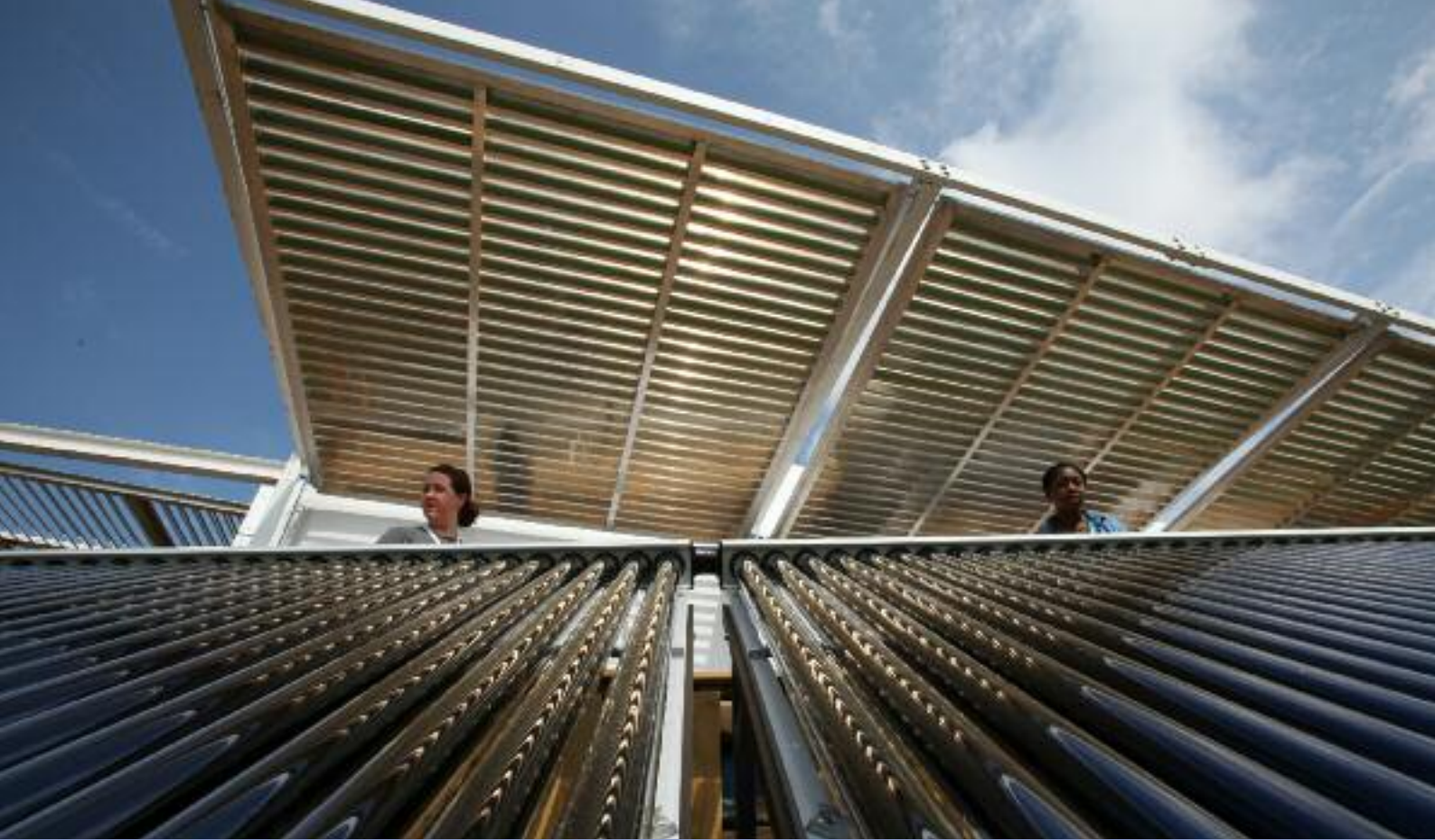
Florida International University's solar thermal collector system. Photo: © Stefano Paltera/U.S. Department of Energy Solar Decathlon
