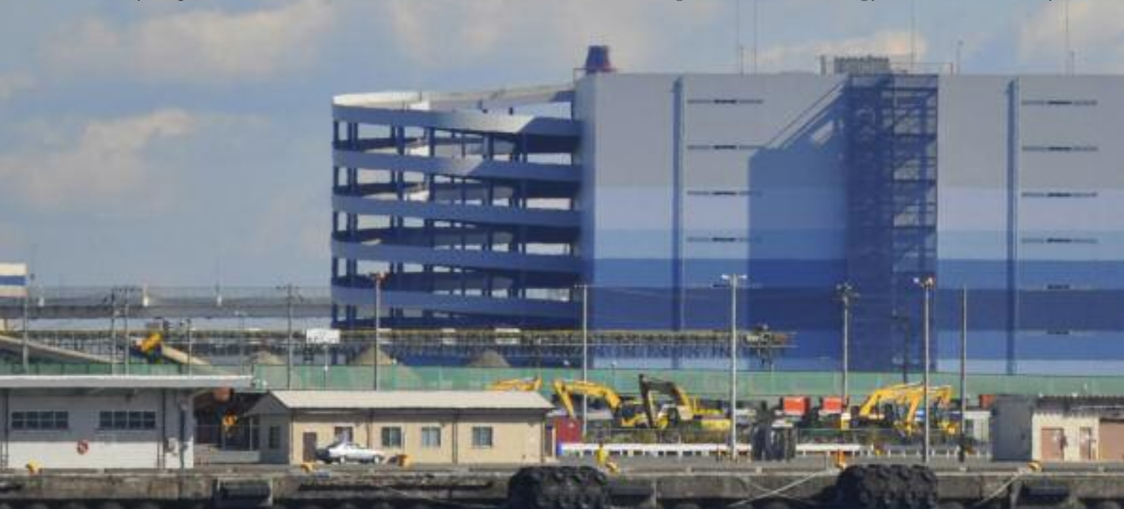
Yokohama Power Station. Photo credit: ISTOCK
