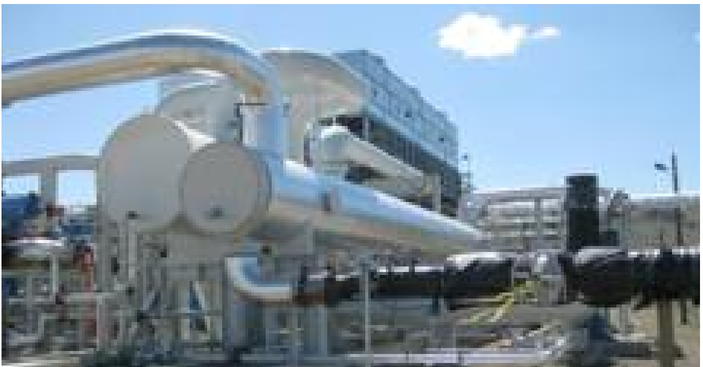
According to the Geothermal Energy Association, two small geothermal energy plants came online in the U.S. in 2014, including this one in Paisley, Oregon. Photo: © Surprise Valley Electric.
