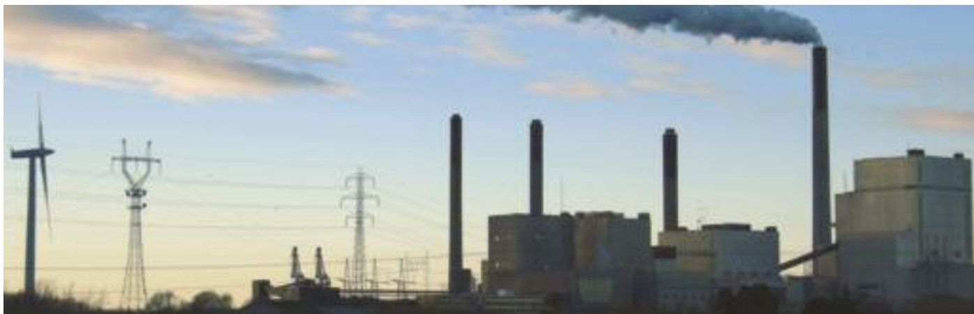
Nordjyllandsværket Power Station boasts the world's most efficient coal use.
