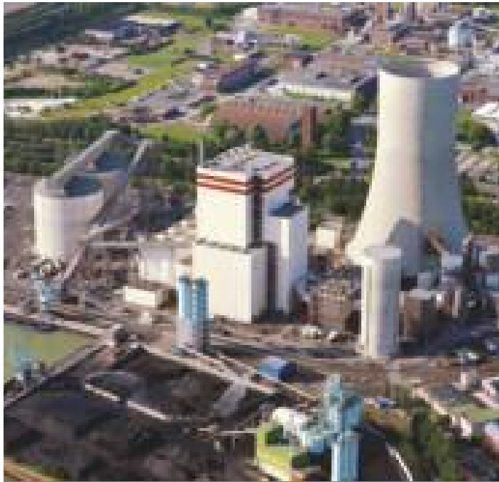
Kohlekraftwerk Lünen power plant Photo: © Trianel
