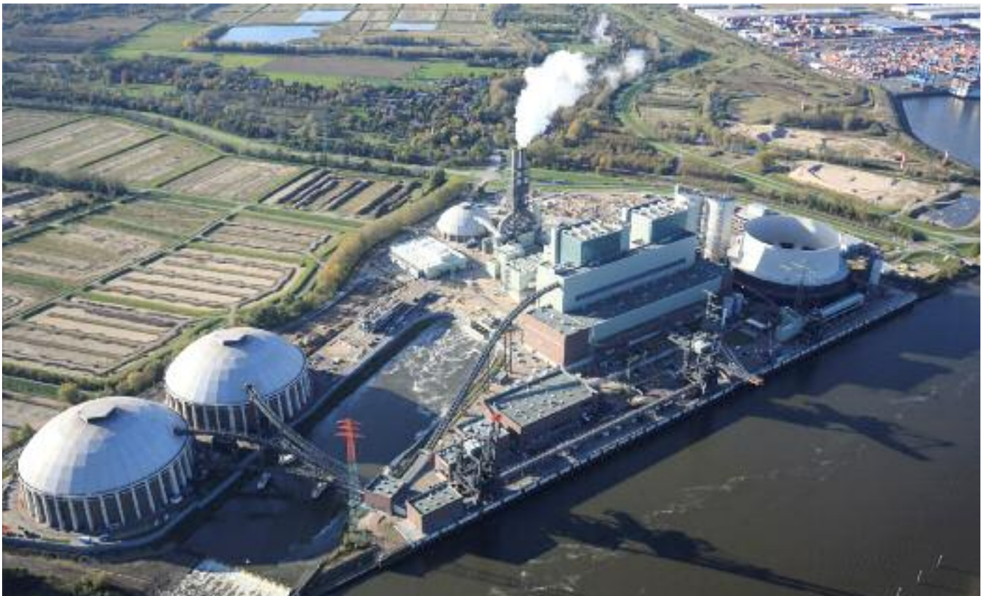
Moorburg (Germany): in late February 2015 regular operation of the first of the two units began. Photo: © Vattenfall.
