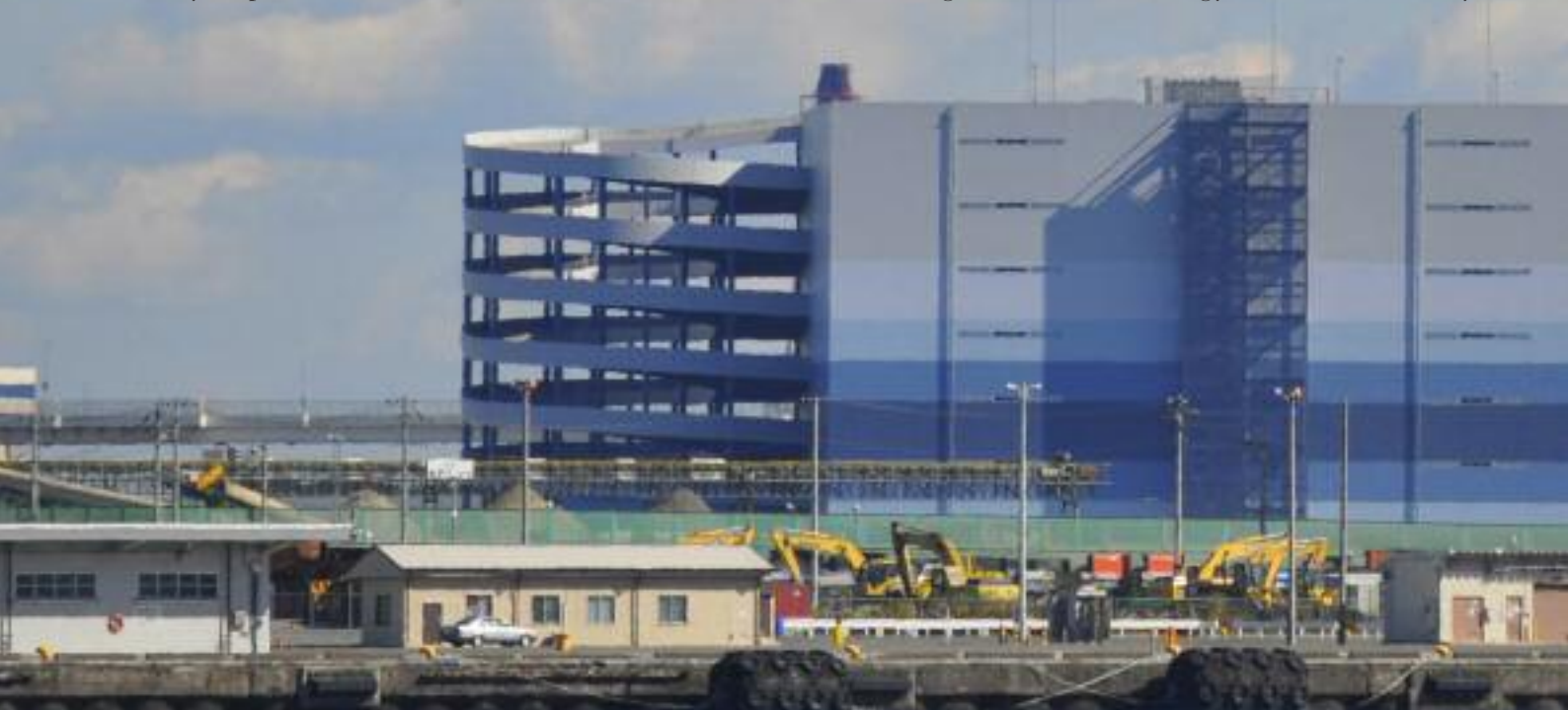
Yokohama Power Station. Photo credit: ISTOCK
